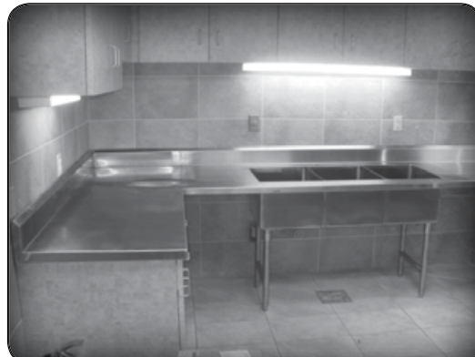
Kitchen Area AFTER
